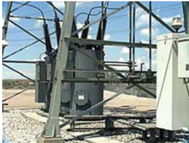
Oil circuit breaker
