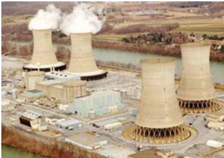
Nuclear Power Station
